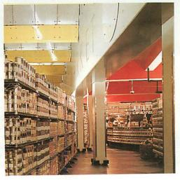
built in four distinct phases between 1860 and 1970. In the 70s intervention a dramatically over-structured series of triangular steel lattice beams was installed to roof over a lightwell which provided the principal escalator circulation.
